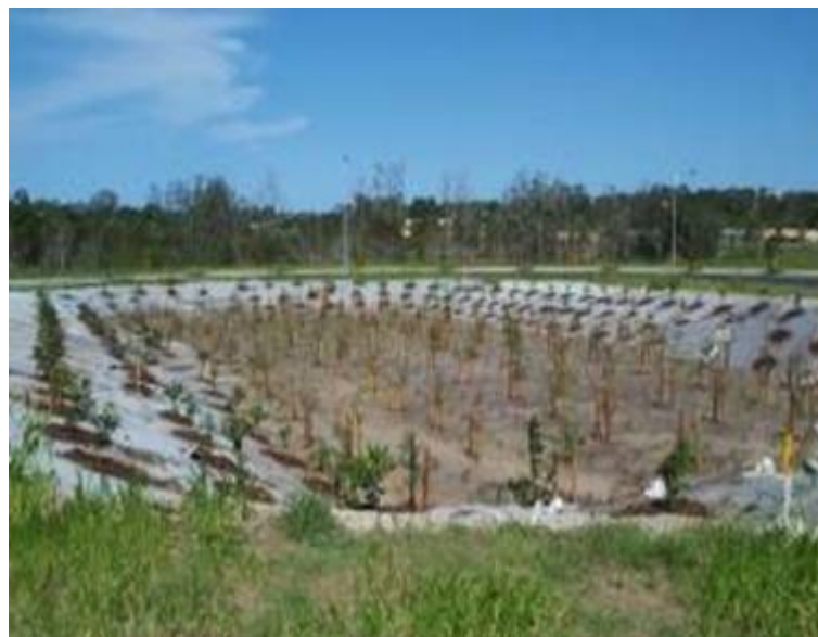
Figure SC6.4.10.23 - Plant Establishment Period in Bioretention Basin
