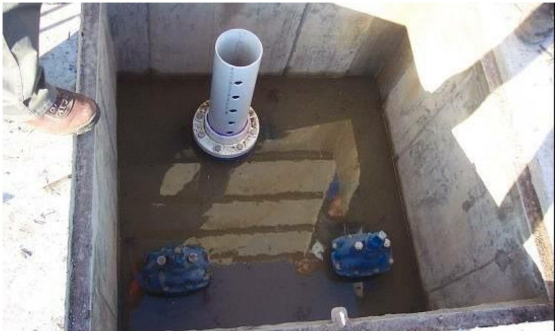
Figure SC6.4.10.38 - Macrophyte Zone Outlet Arrangement
