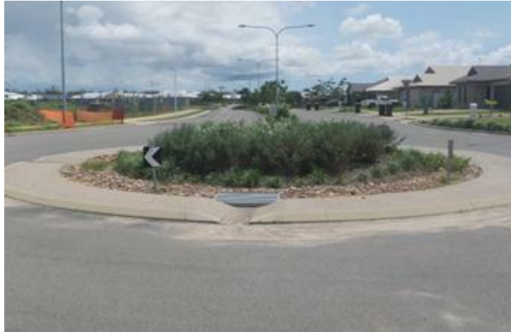
Figure SC6.4.10.17 - Bioretention Basin Within Roundabout at Kalynda Chase Development, Bohle Plains
