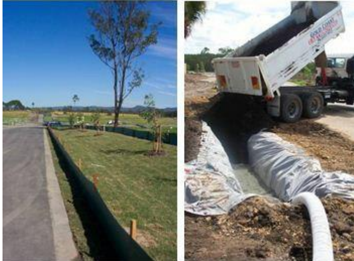
Figure SC6.4.10.14 - Bioretention Swale Functional Installation
