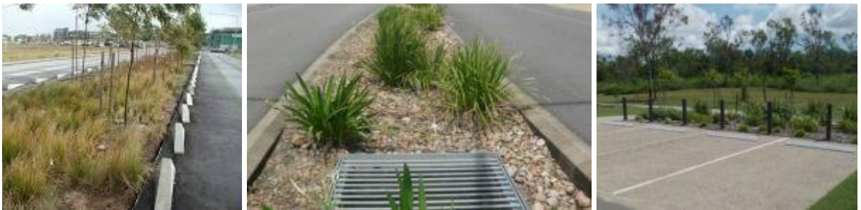
Figure SC6.4.10.5 - Kerb Arrangements with Breaks and Flush Kerbs to Distribute Inflows onto Bioretention Swales and Prevent Vehicle Access
