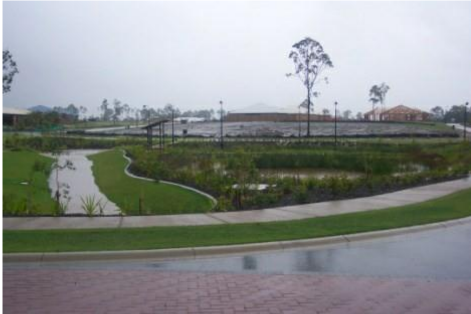
Figure SC6.4.10.47 - Constructed Wetland Sediment and Erosion Control Operation
