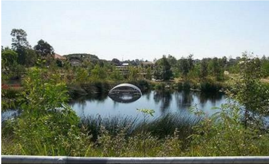
Figure SC6.4.10.31 - Inlet Zone of a Constructed Wetland in Brisbane
