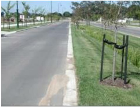
FigureSC6.4.10.6 - Flush Kerb Without Set Down, Showing Sediment Accumulation on Road
